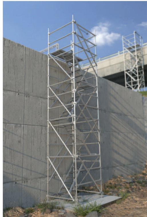
Staircase tower for construction site access
